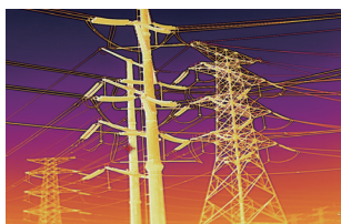
Electric Routine Inspection
